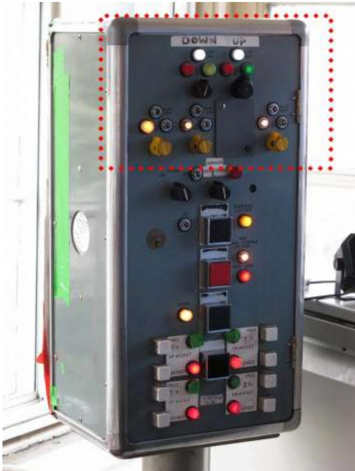
The crossing is kept locked until the train has passed, and only then can the Crossing Keeper raise the barriers.
