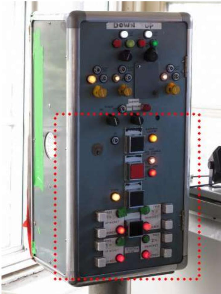
Once the barriers have closed, the Crossing Keeper makes a thorough final check that the crossing is clear and then uses the switches at the top of the control panel to clear the relevant signal or signals to Green. In an emergency the signals can be set back to Red by either the Crossing Keeper at Foxton or the Signal Box at Cambridge.
