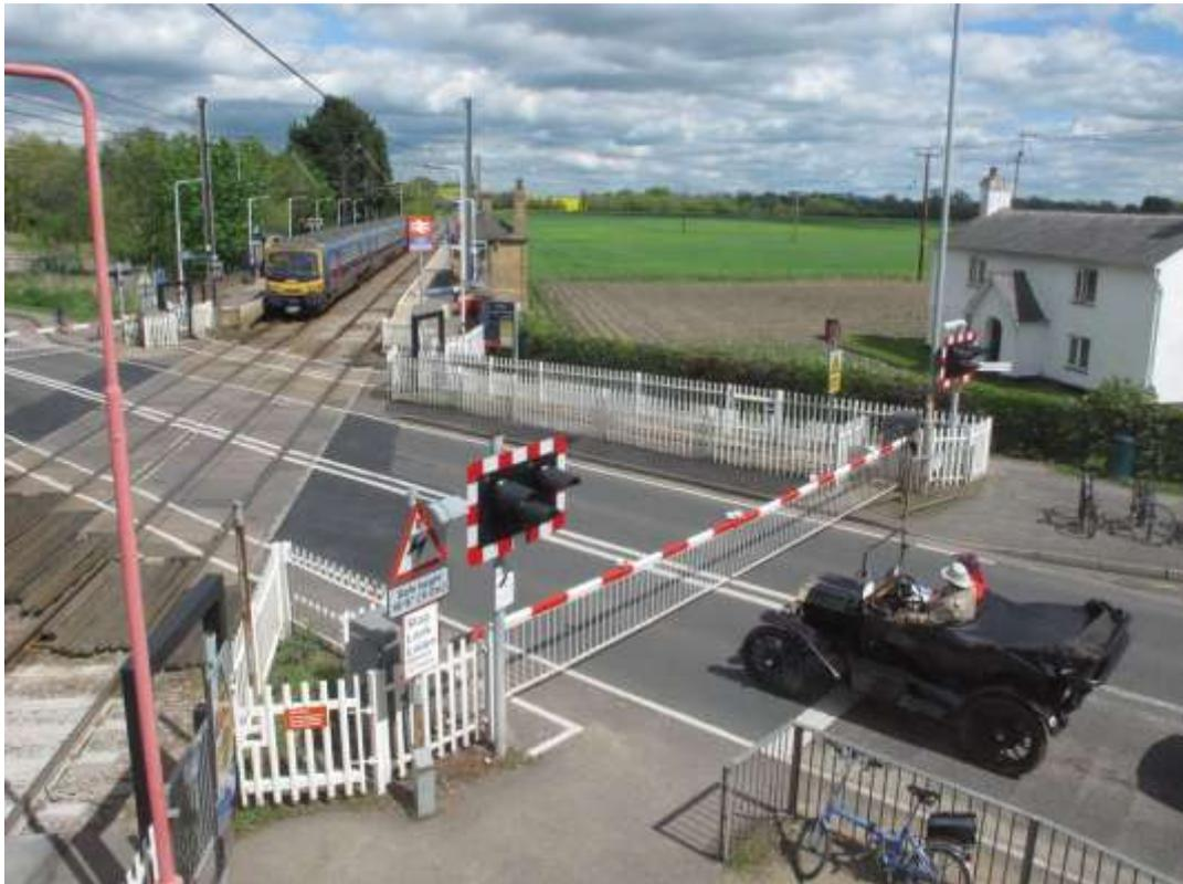
A video camera continuously records the crossing to provide evidence in the case of an incident or misuse of the crossing. Several days of video are stored.
